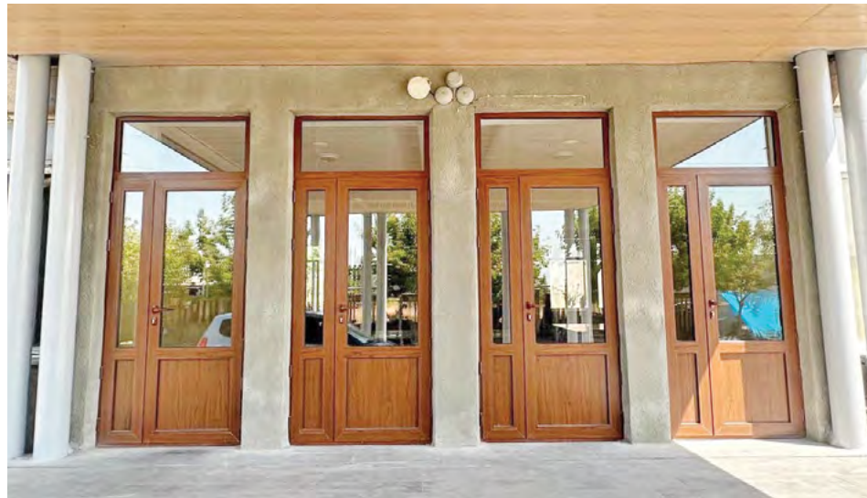
New entrance doors installed in August 2025
