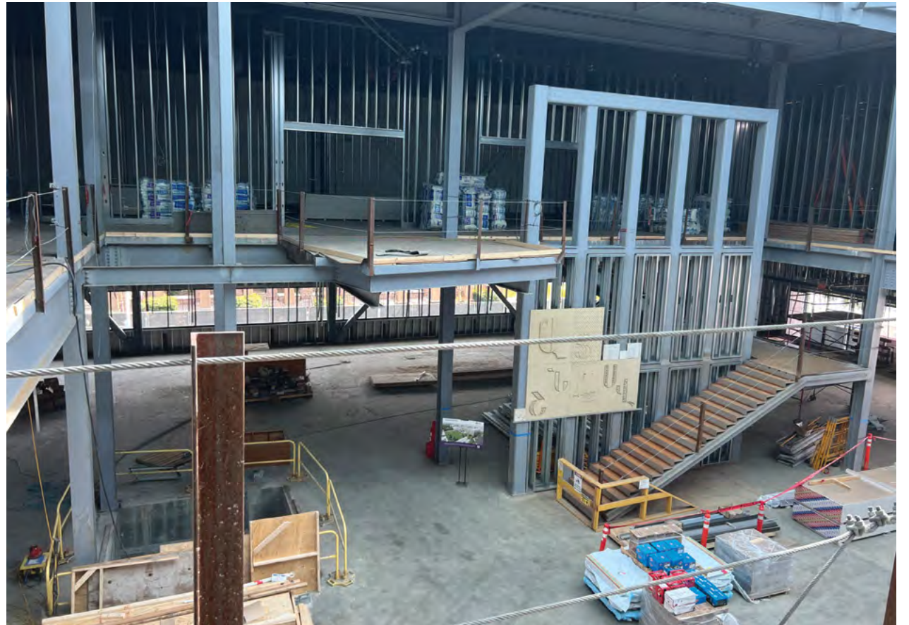
The first and second floors under construction (photo Aram Arkun)
