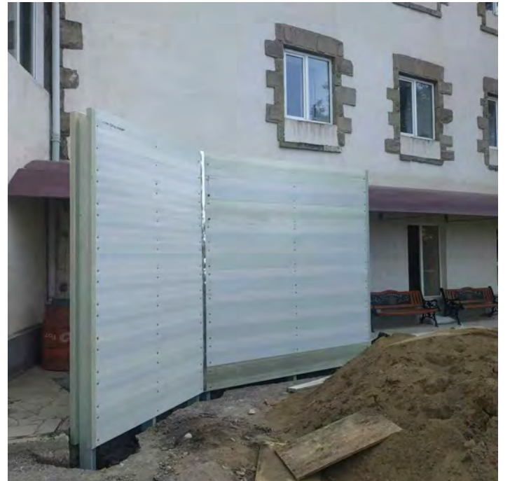
Sand-filled defensive barrier installed at Aygehovit secondary school by the Pahapan Foundation (courtesy of Pahapan Foundation)
