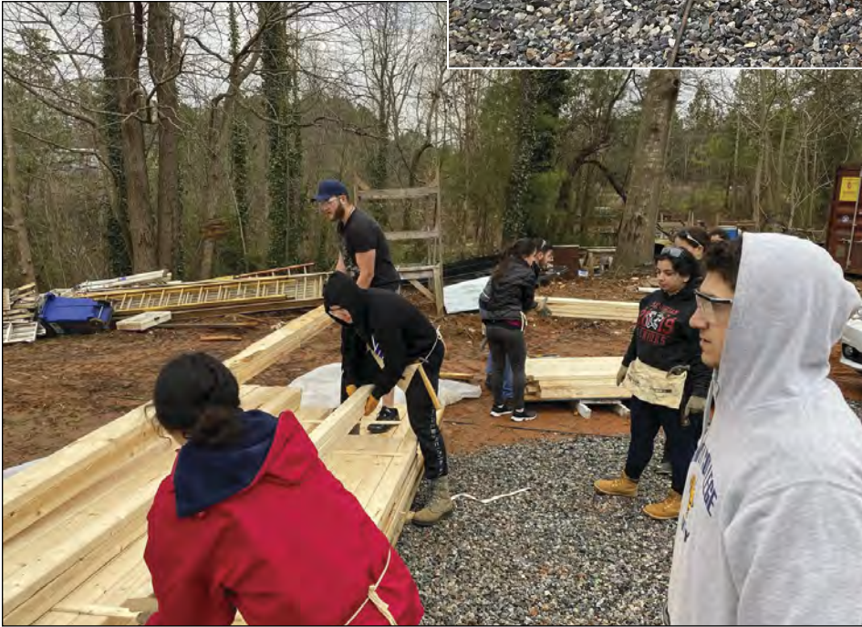
Hard at work with construction materials
