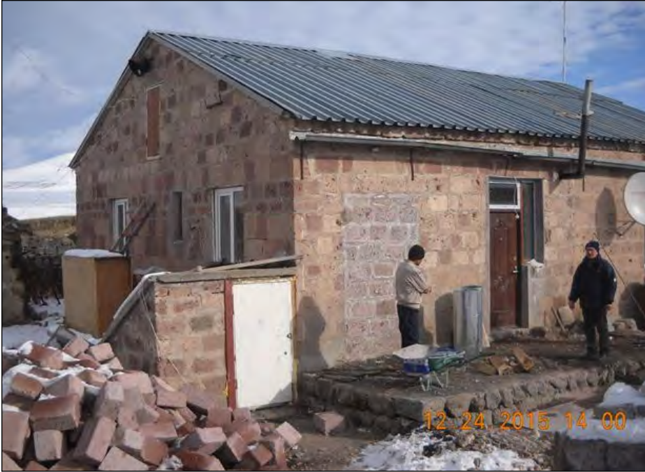
The Tevosyan home under construction
