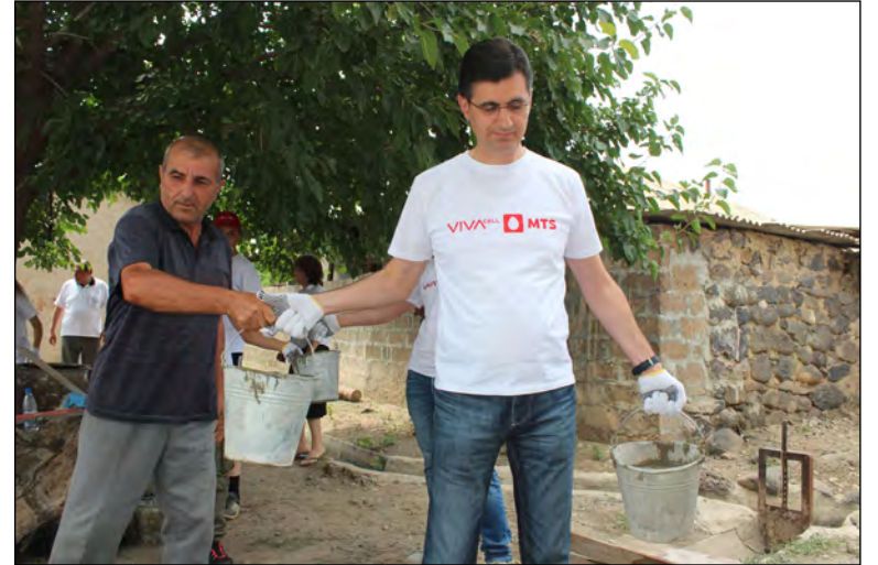
VivaCell’s Ralph Yirikian helped out with the construction.
