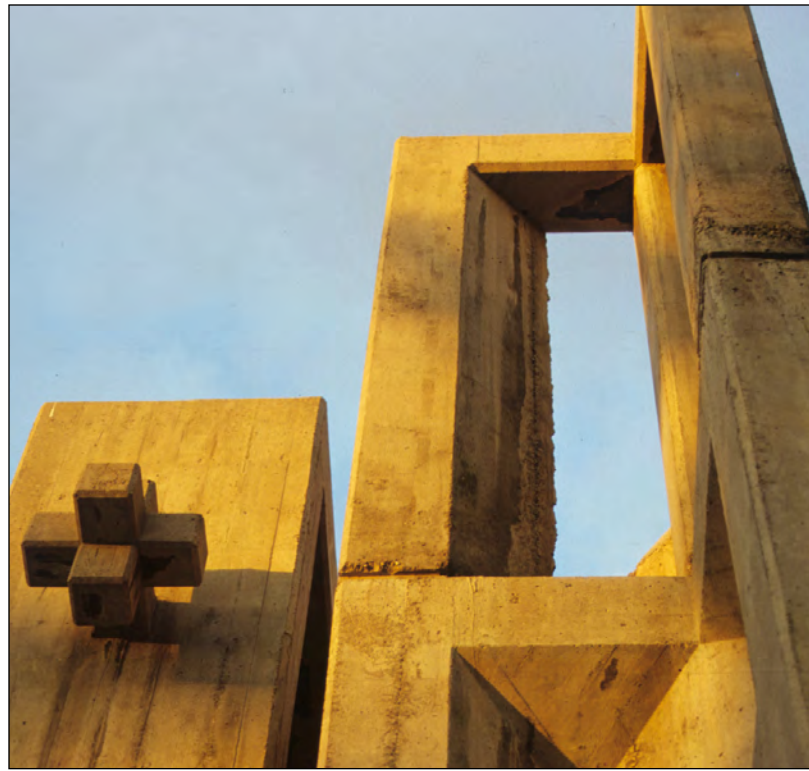
Detail of Holy Cross Chapel, Ararat Stadium complex, Tehran, Iran
