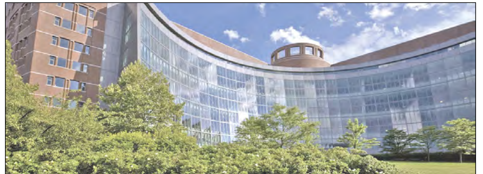
The John Joseph Moakley Courthouse overlooking Boston Harbor
