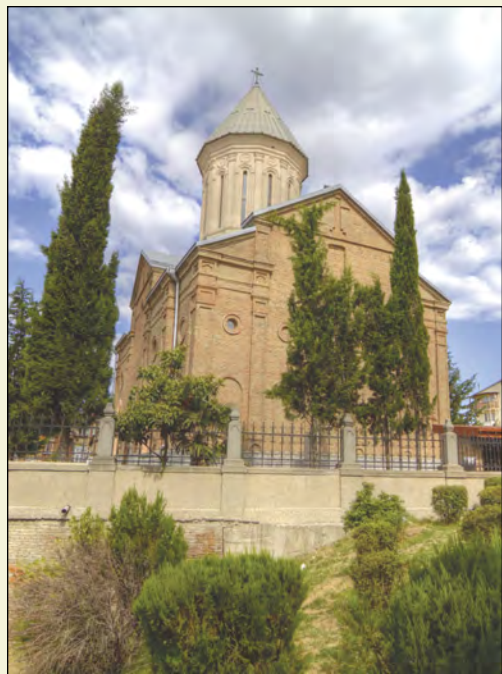
Surb (Holy) Echmiadzin Church in Tbilisi
