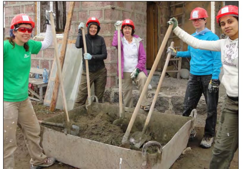
Volunteers help construct a home.
