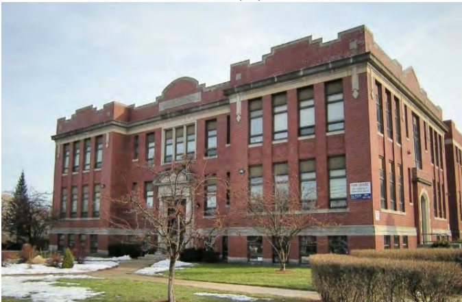
Parker School Building, Location of Law Offices of Gregory H. Arabian & Associates, LLC
