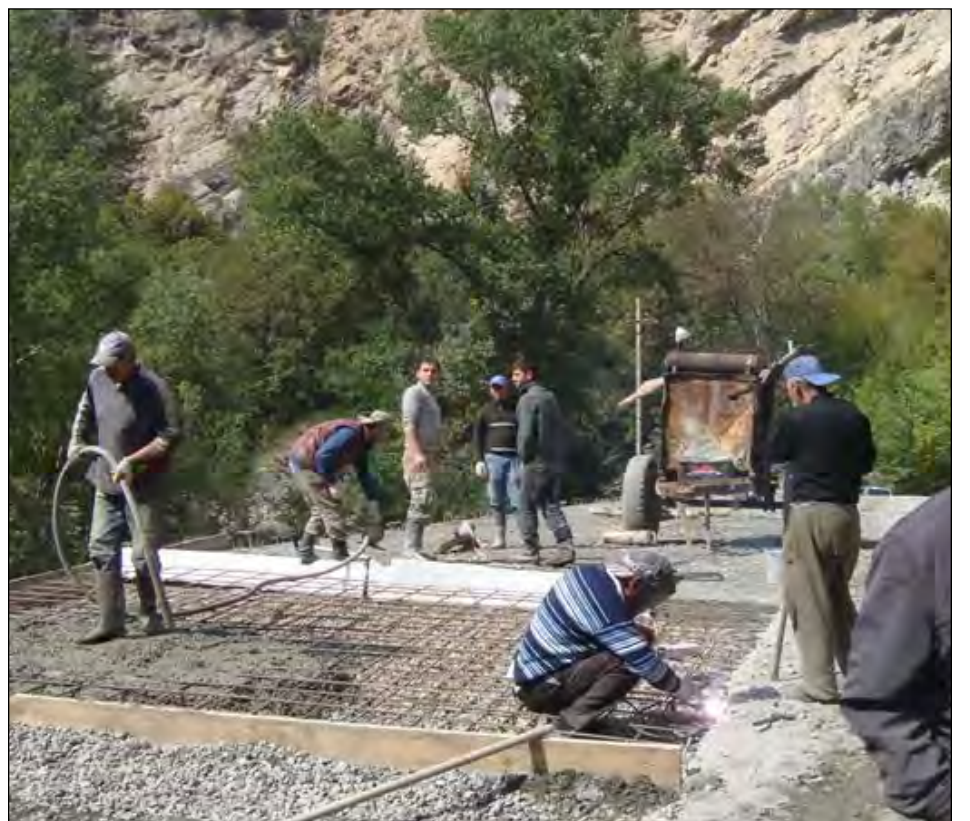
Construction crew actively building the road
