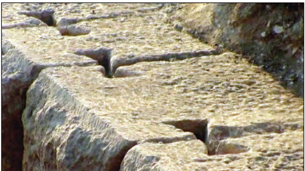
“Tigranakeri” : A detail of the “swallowtail” technique of Classical Armenian masonry
